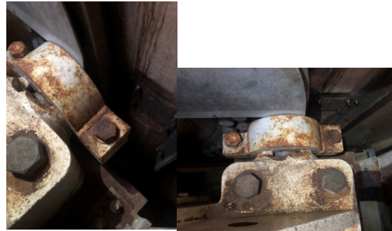
Fig. 18. Final implementation of redesigned hub pin lock mechanism on the operational wind turbine.
