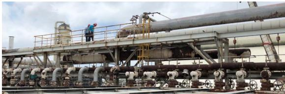
Fig. 2. A practical fractionator overhead vapor line.
