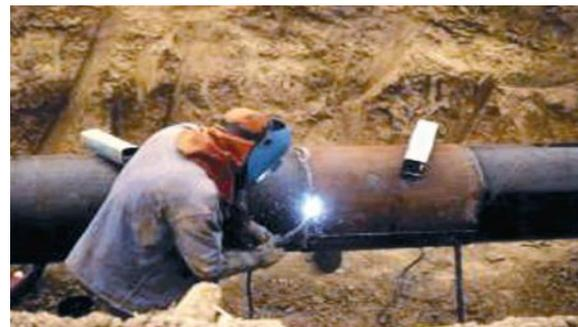
Fig. 8 Half-shell welding operation (A. Benlekhal, 2010)
