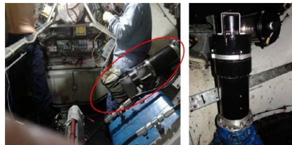
Fig 16. Pitch motor: old motor(left)/new motor(right)
